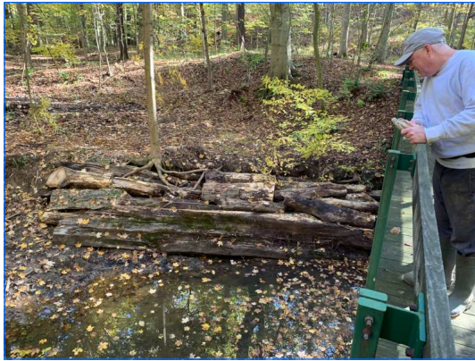
Trail Crew volunteer Don Voorhees views the logs placed for erosion control on the east bank of the creek.
