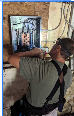
Hal Goodwin makes final connections.
