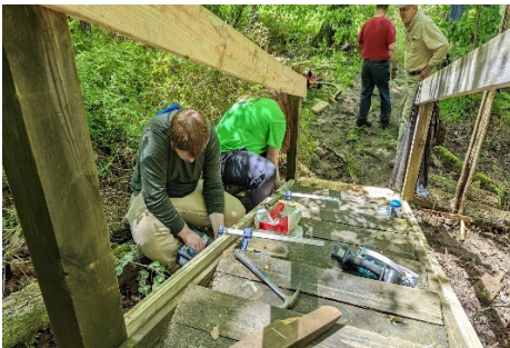
Repairing windfall damage to a stairway in the Aurora Sanctuary
