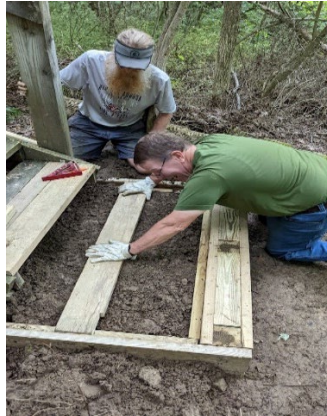
Repairing windfall damage to a stairway in the Aurora Sanctuary
