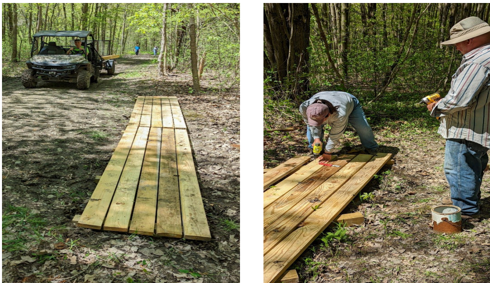
Creating small boardwalks to bridge muddy trail areas in the west Novak Sanctuary
