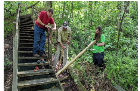
Repairing windfall damage to a stairway in the Aurora Sanctuary
