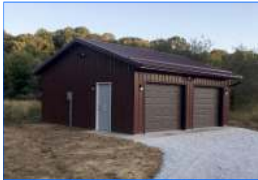
New storage shed at Hach-Otis Sanctuary.
